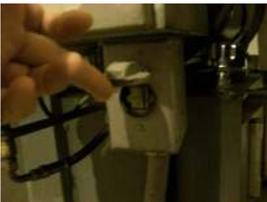
Replaced “project installed” cutoff switches so that they could be locked-out
