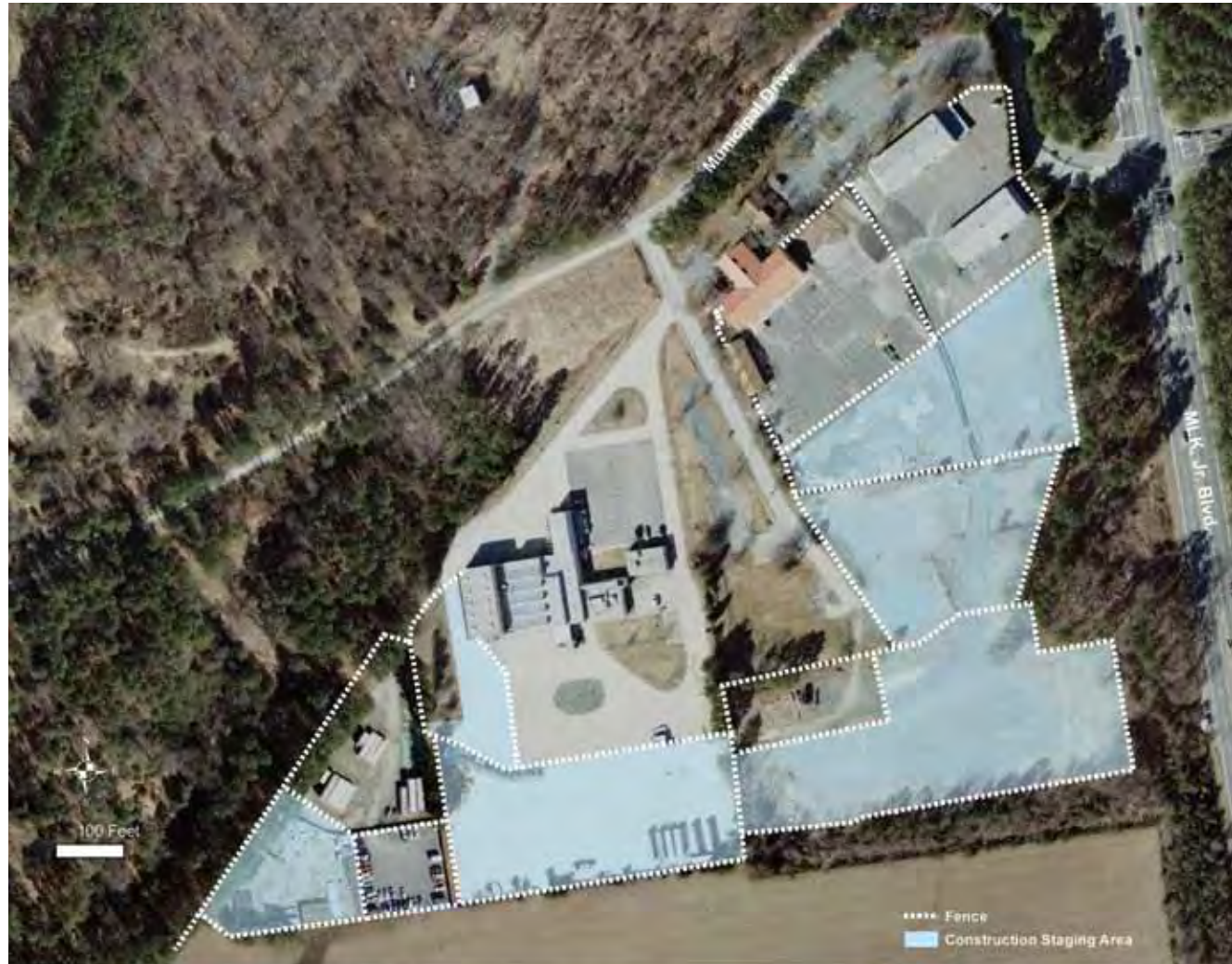
Site storage and construction staging areas
