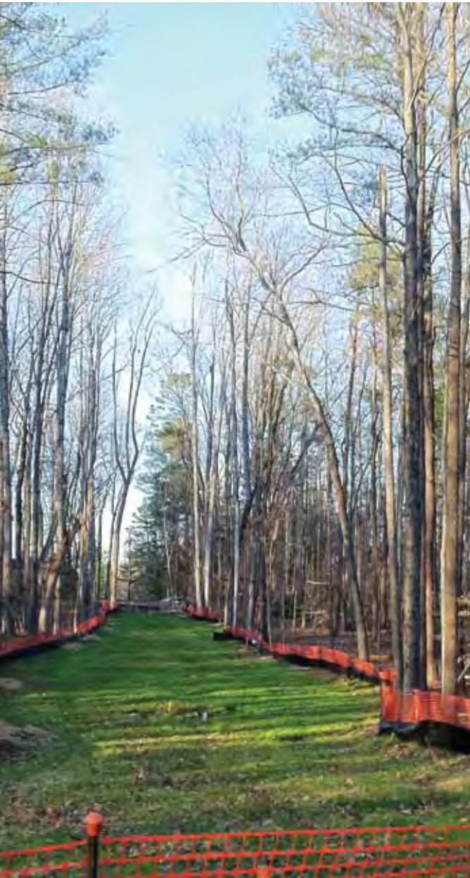
The electric ductbank construction corridor
