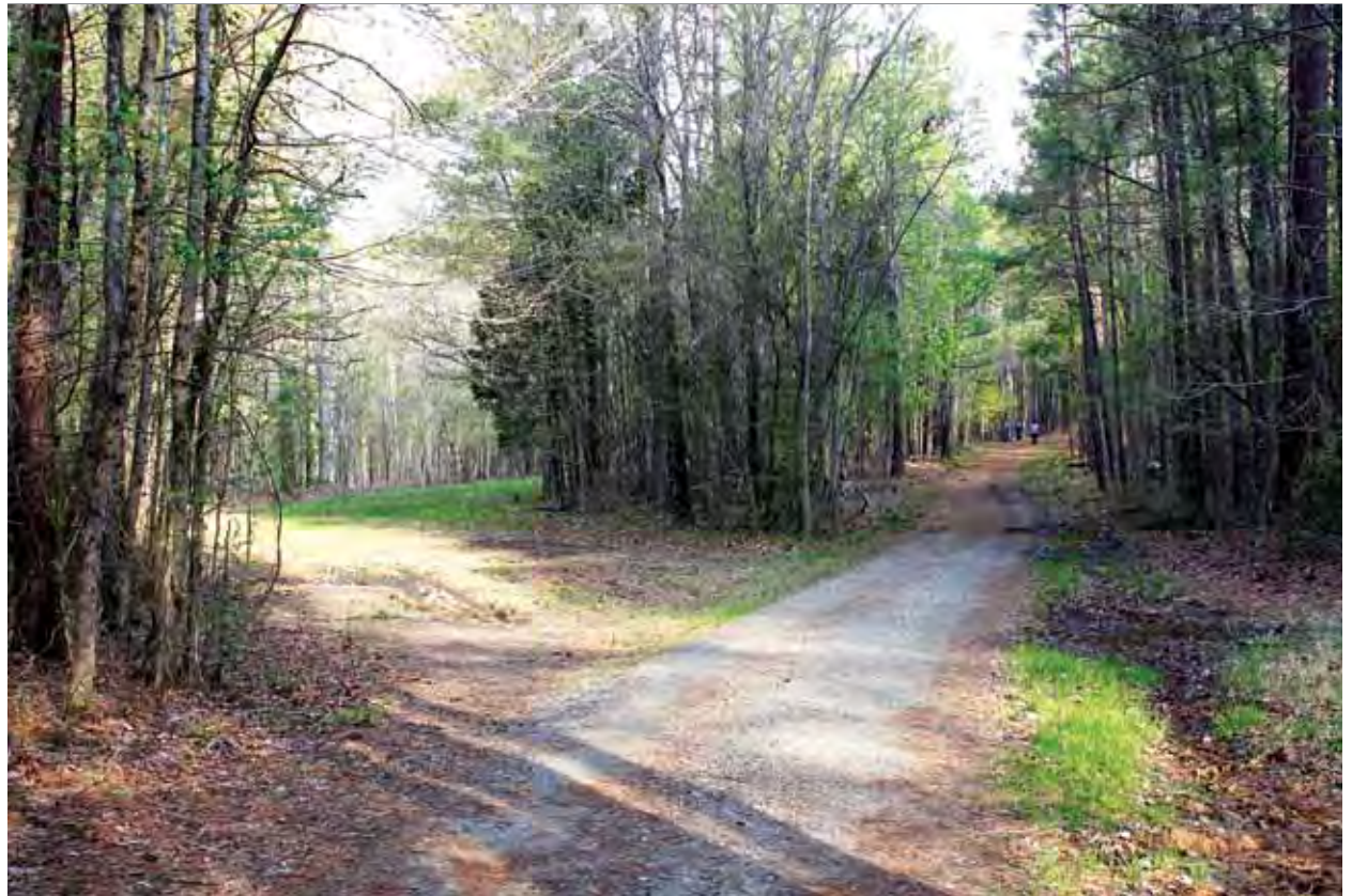
Pumpkin Loop Service Road at PSNC corridor
