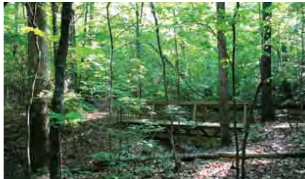
Carolina North Forest bridge
