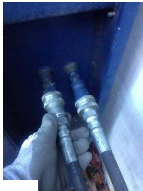
Hydraulic hose connected [Figure 11]
