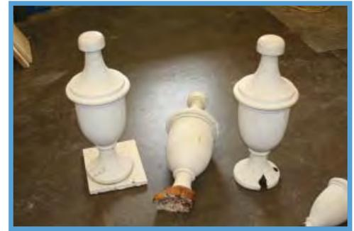
**Carpenters can repair most of the cupola's decorative finials, but one is so damaged a new one will be constructed.**
