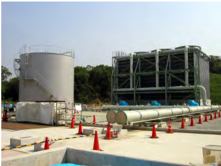
Water tank and cooling tower
