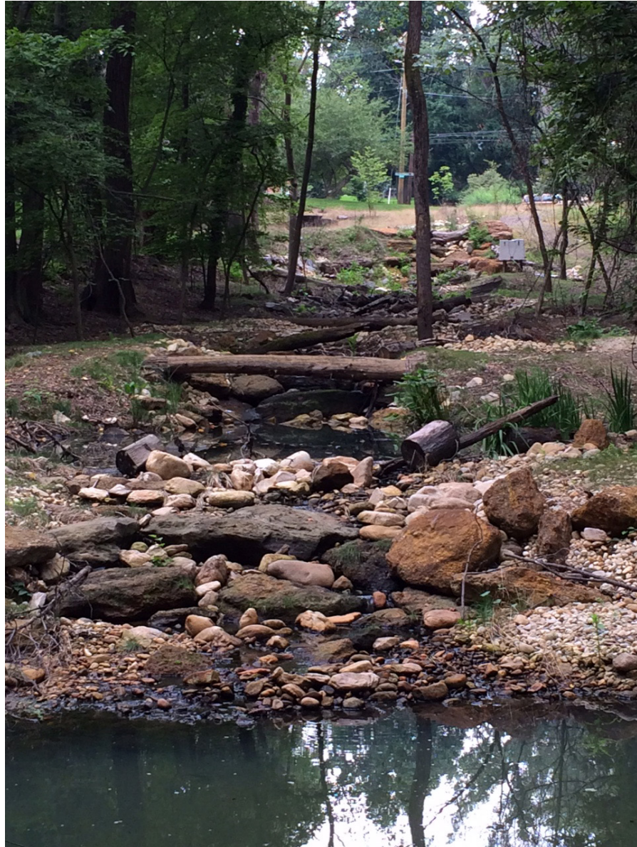
Example of stream channel restoration with improved sediment and pollutant processing of stormwater runoff
