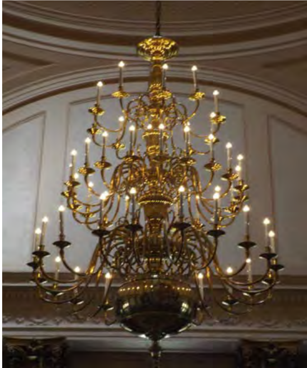
Wilson Library's chandeliers incandescent lamps replaced with LED lamps
