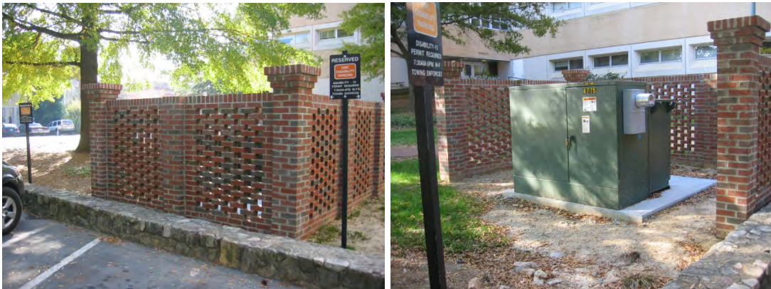
The pictures above show an example of a 3-sided screen wall located at Hamilton Hall. The fourth side is open for access to utilities.
