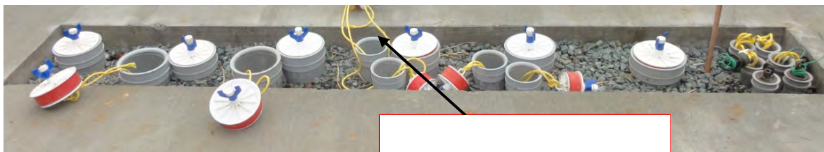
Figure 3: Electrical Conduits End Point Stubbed Up with End Bells and Plugs.
