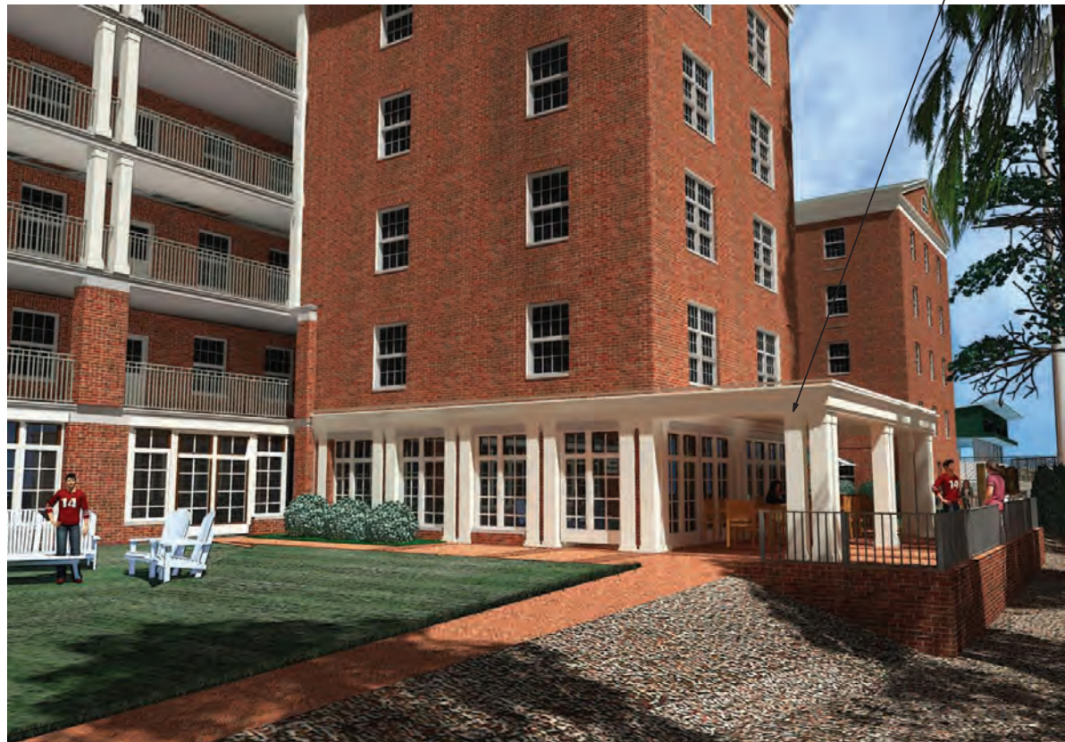
SOUTH WEST VIEW
